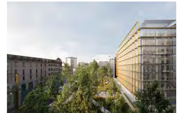
OBR - Bassi Business Park, Milano
